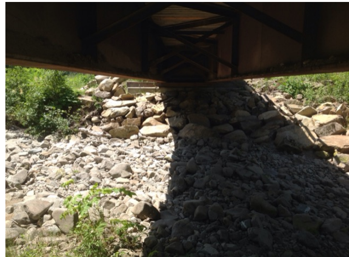
Right Bank Abutment when facing downstream
