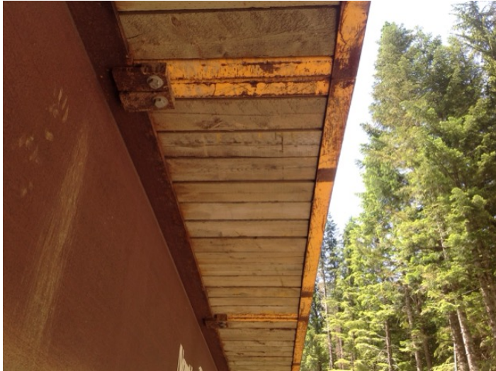
timber deck panels with HSS rails
