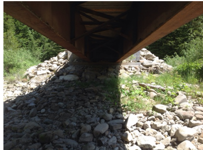
Left Bank Abutment when facing downstream
